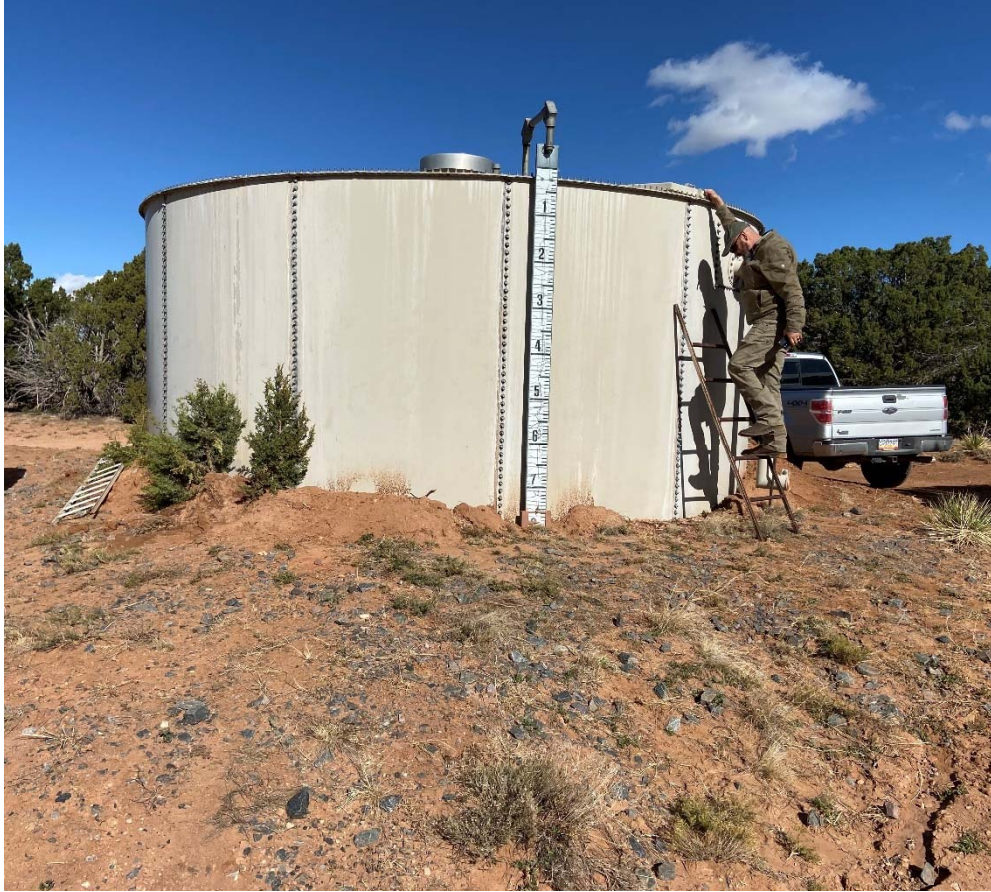
Figure 11 – Bolted Steel Tank
